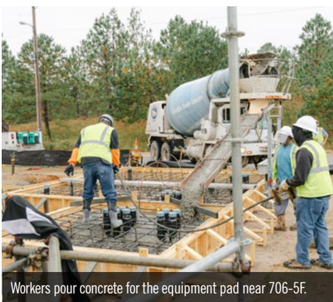
Workers pour concrete for the equipment pad near 706-5F.
